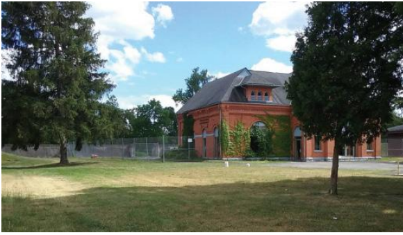
Old Water Building at Elmira
